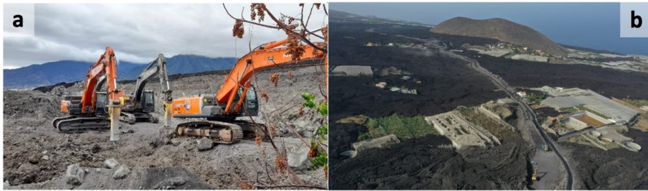
Figure 11: Excavators removing volcanic material for the opening of roads and paths.
