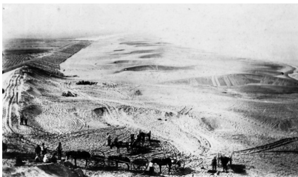
Figure 5. Dune fixation work in St. Martí d'Empúries, l'Escala, around 1896. In the background, barchanoid morphologies perpendicular to the coast, caused by the tramontane, can be observed. Source: Josep Esquirol Collection, Municipal Archives of l'Escala.
