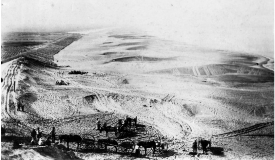
Figure 5. Dune fixation work in St. Martí d'Empúries, l'Escala, around 1896. In the background, barchanoid morphologies perpendicular to the coast, caused by the tramontane, can be observed. Source: Josep Esquirol Collection, Municipal Archives of l'Escala.
